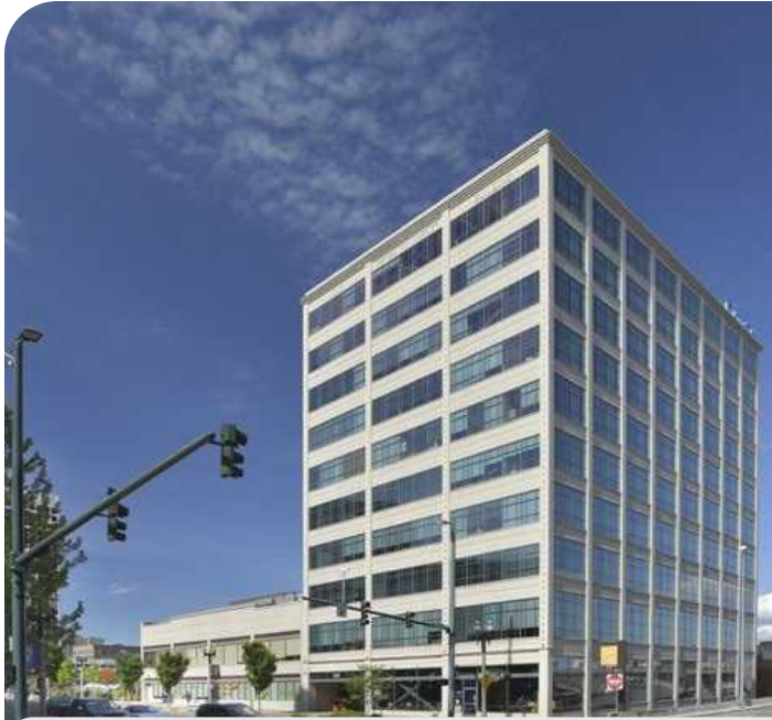
BUILDING FROM 14 TH & PACIFIC AVENUE
