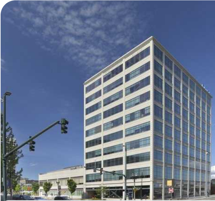
BUILDING FROM 14 TH & PACIFIC AVENUE
