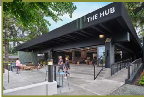
20' NANO WALL PROVIDING INDOOR/OUTDOOR CONNECTION
