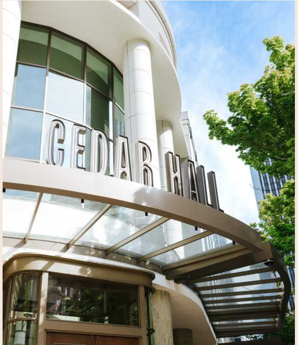
Entrance at 5th and Pike
