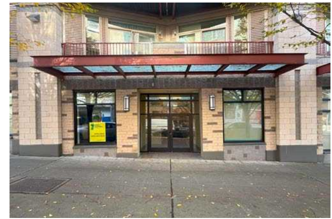
ENTRANCE FROM NW 57 TH STREET
