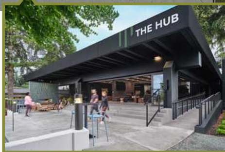
20' NANO WALL PROVIDING INDOOR/OUTDOOR CONNECTION
