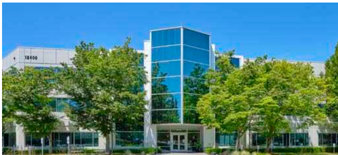
Building C | 18400 NE Union Hill Rd Full Building: 33,298 - 99,945 SF Available
