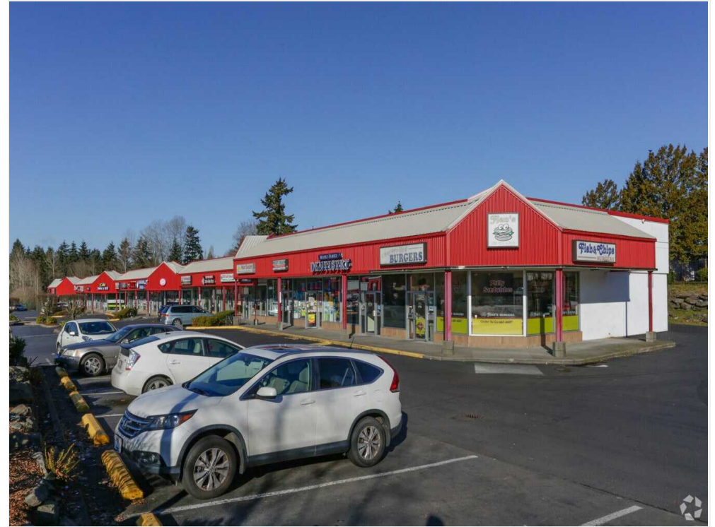
2120-2324 SW 336th St - Twin Lakes Shopping Center
