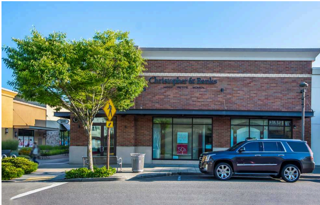
SUITE 105 IN BUILDING THIRTEEN
