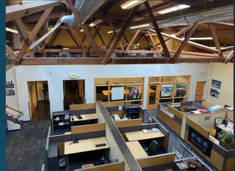
View looking west from Mezz
