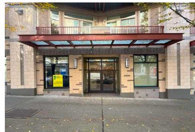
ENTRANCE FROM NW 57 TH STREET
