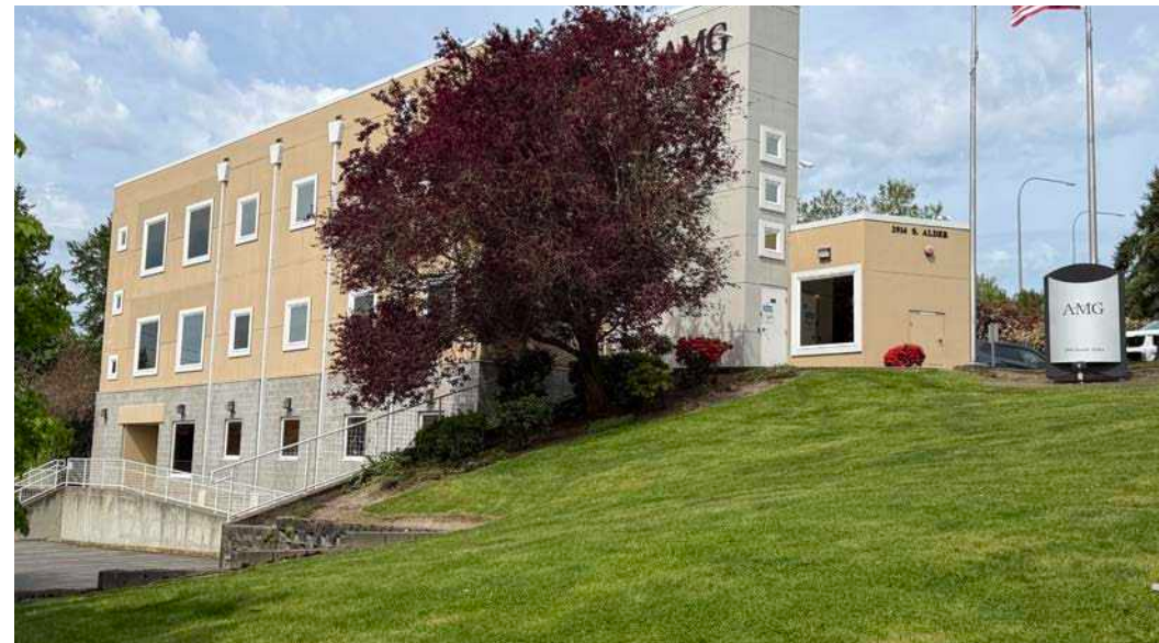
LOWER LEVEL ENTRANCE
