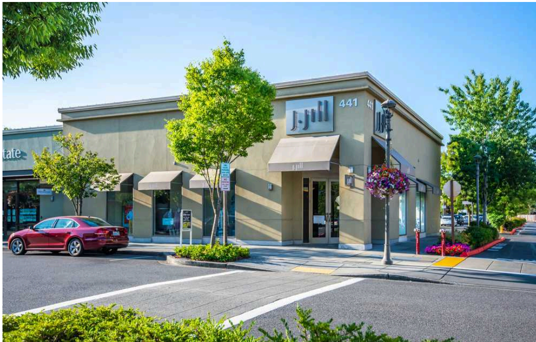
SUITE 105 IN BUILDING FIFTEEN
