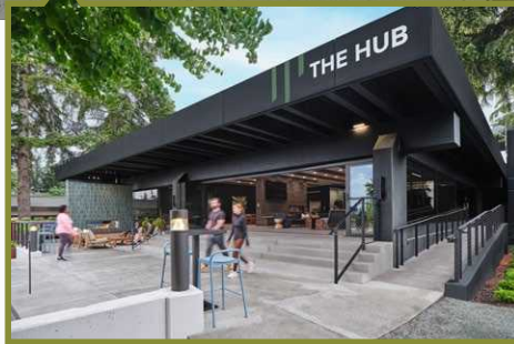
20' NANO WALL PROVIDING INDOOR/OUTDOOR CONNECTION
