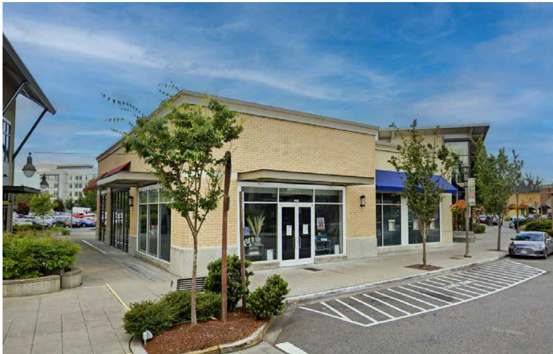
SUITE 102 IN BUILDING TWO
