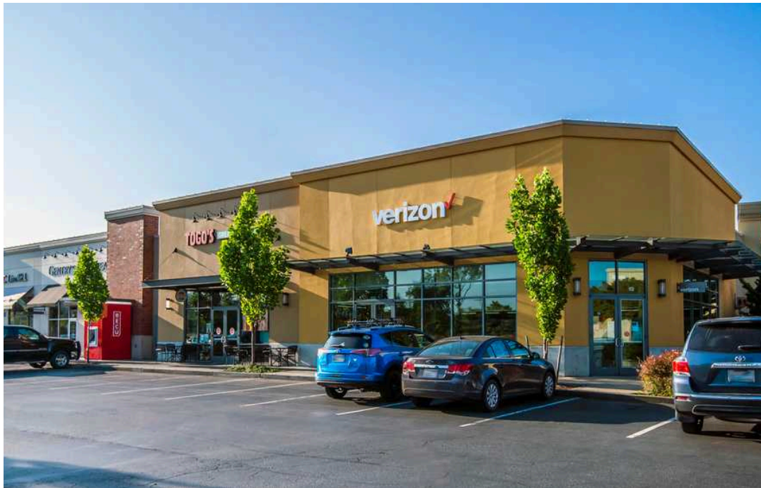
SUITE 112 IN BUILDING THIRTEEN
