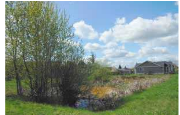
A residential stormwater retention pond.
