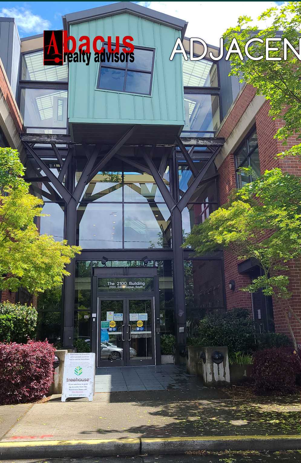
E VIEW OF 2100 BLDG FROM 24TH AVE S
