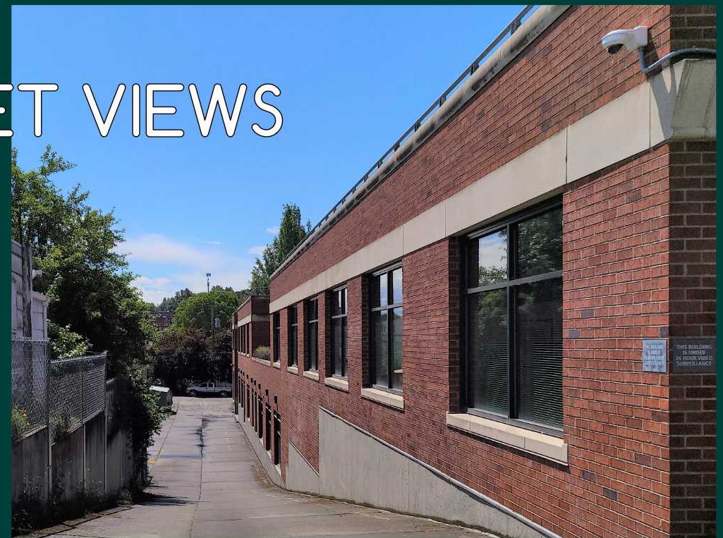
S VIEW OF CONCRETE-PAVED CITY ALLEY FROM S HILL ST
