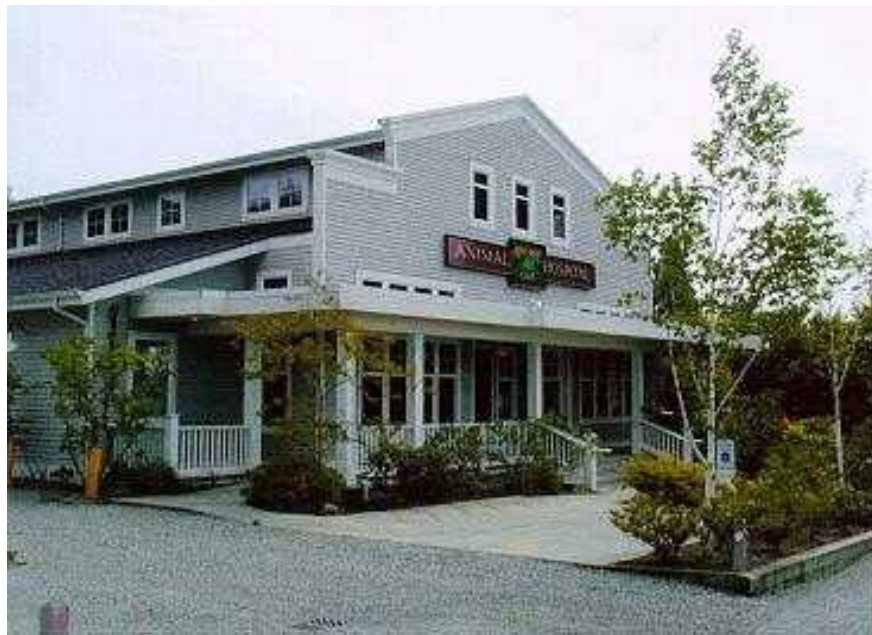
Figure IV-2. This contemporary interpretation of traditional architecture would be appropriate in all three downtown design districts. The simple gable form, traditional siding, appropriate sign, welcoming porch, and transparent front façade make it pedestrian friendly and consistent with the town's identity. Note how the multi-paned windows, porch railing, and porch column details all add a simple grace and human scale without being overly ornamental. The colors, light gray with white trim, are appropriate. The landscaping also enhances the development's qualities.
