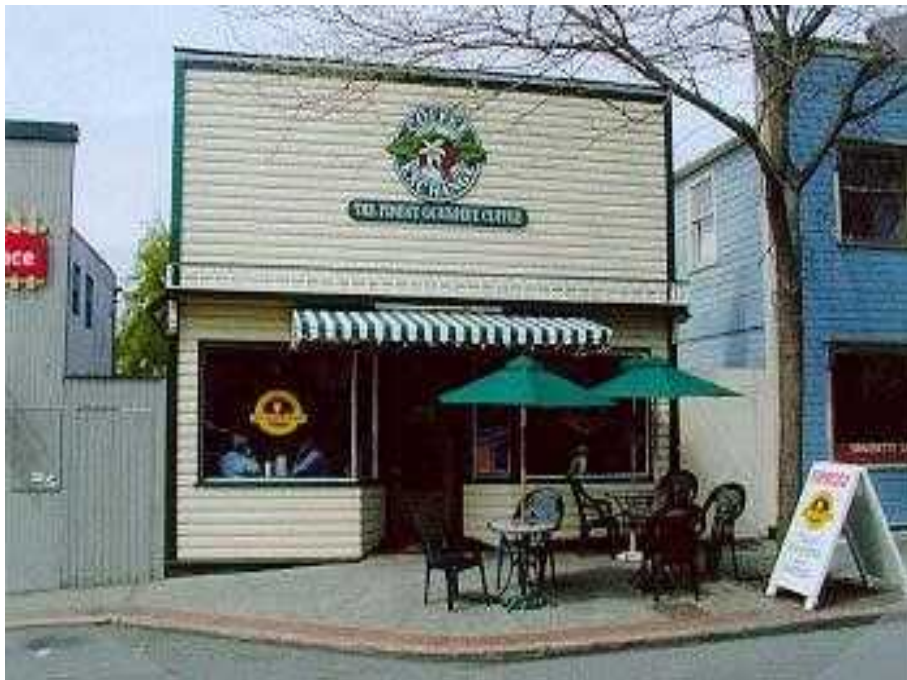
Figure IV.B.1.(a). The front of this tiny coffee shop features many pedestrian-oriented elements, including weather protection, decorative lights, modest but effective ornamentation, traditional siding, recessed entry, and large display windows. Note the outdoor table and chairs. Add the smell of fresh brewed coffee and you have a customer magnet, not only for the coffee shop, but neighboring businesses as well.
