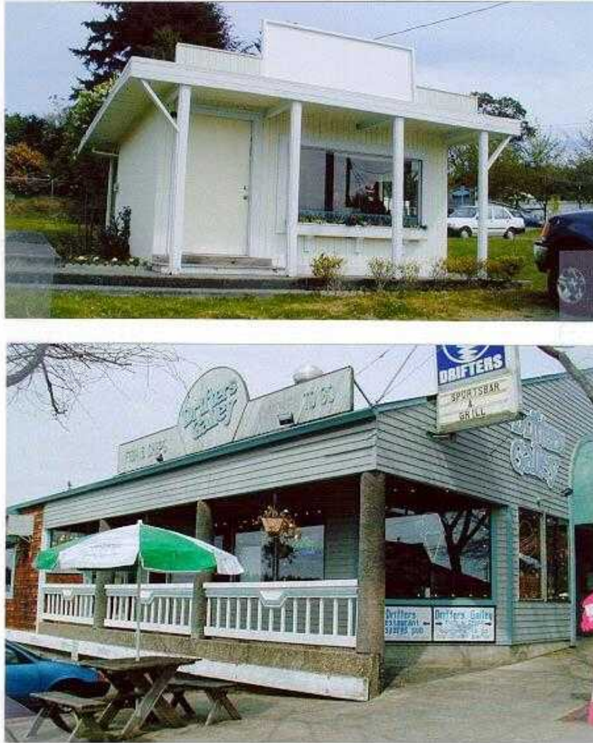
Figure IV.B.1.(b).1. Two examples of porches. Though simple, the top porch adds a bit of comfort and protection to an otherwise plain façade. The bottom example illustrates how a covered entryway can be effectively integrated into building design.
