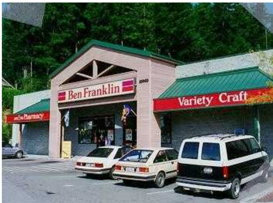
Figure IV.B.1.(d). The Ben Franklin store façade incorporates metal roof arcades and a gabled entryway to add interest and human scale to a concrete masonry unit building.
