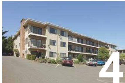
Queensview Apartments 13007-13035 12th Ave SW, Burien
