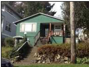
Duplex 4023 1st Ave NE
