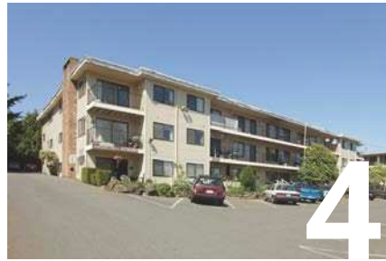
Queensview Apartments 13007-13035 12th Ave SW, Burien
