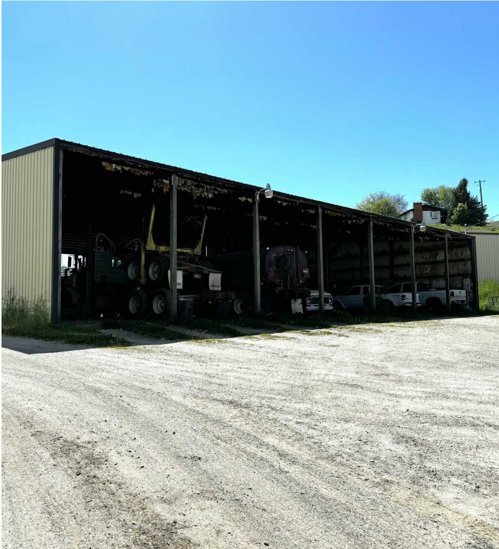
Pole Barn +/- 5,600 SF: 6 Covered bays, perfect for equipment, trucks, or materials
