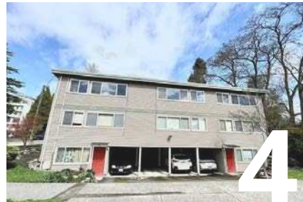
Dorlynn Apartments 8800 Nesbit Ave N, Seattle, WA 98103
