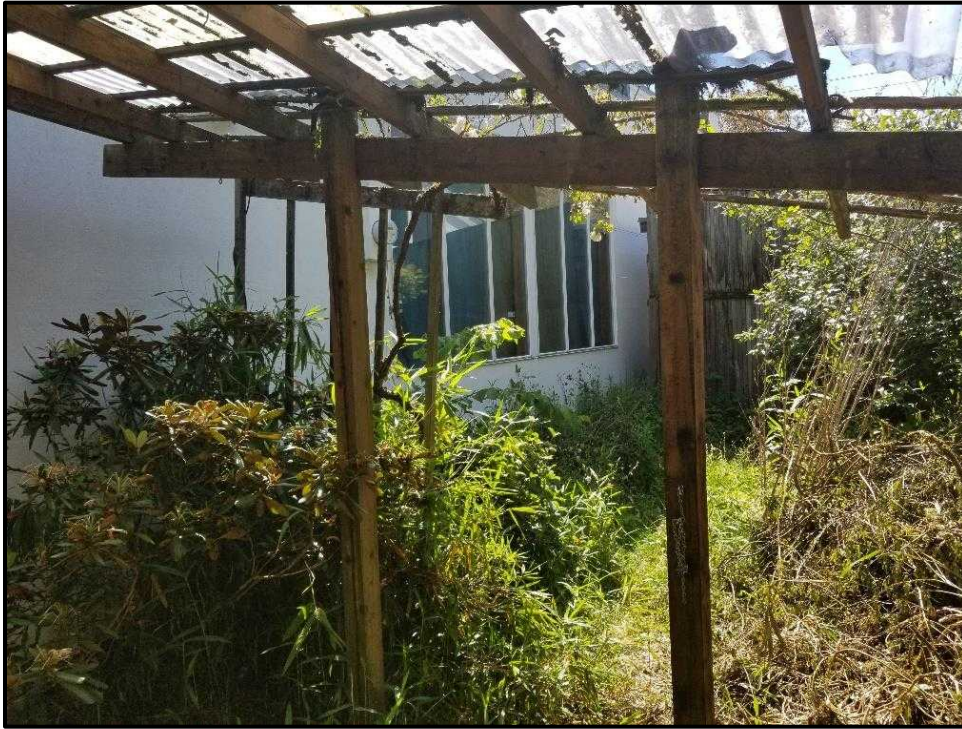
13. View looking at the breezeway between the two buildings.
