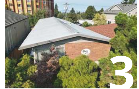
Bruce Apartments 6339 42nd Ave SW
