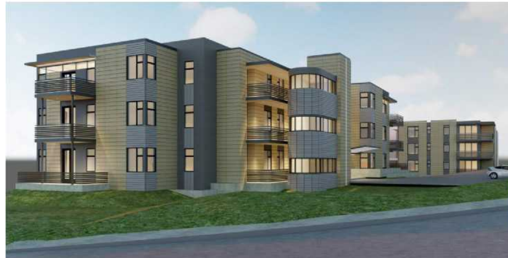
View Looking South
