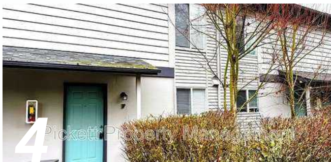
4 HIDDEN COVE APARTMENTS
