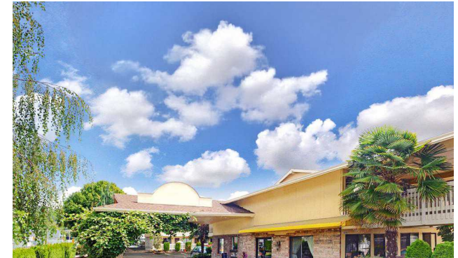
Exterior of Building
