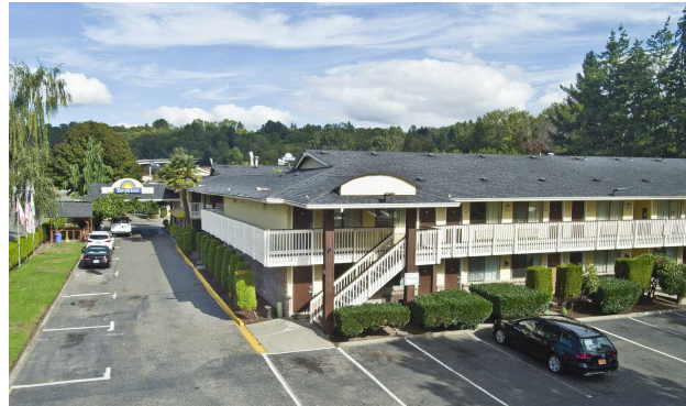
Exterior of Building
