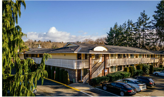
Exterior of Building
