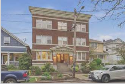
Wiltona Apartments Seattle, WA
