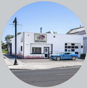
NEW ROOF TO BE COMPLETED PRIOR TO CLOSING
