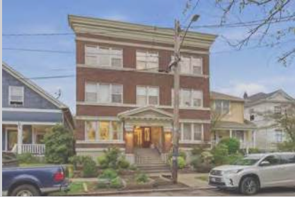
Wiltona Apartments Seattle, WA
