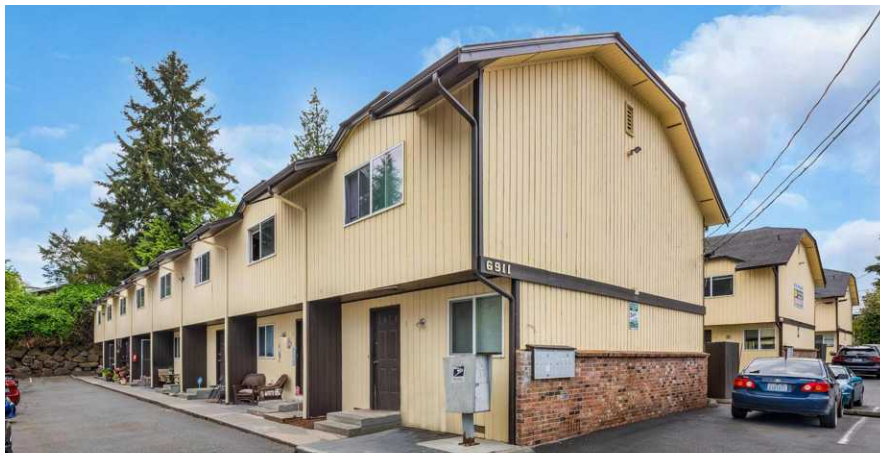
2 Rainier Townhouse Apartments 6911-6921 Rainier Drive, Everett, WA 98203
